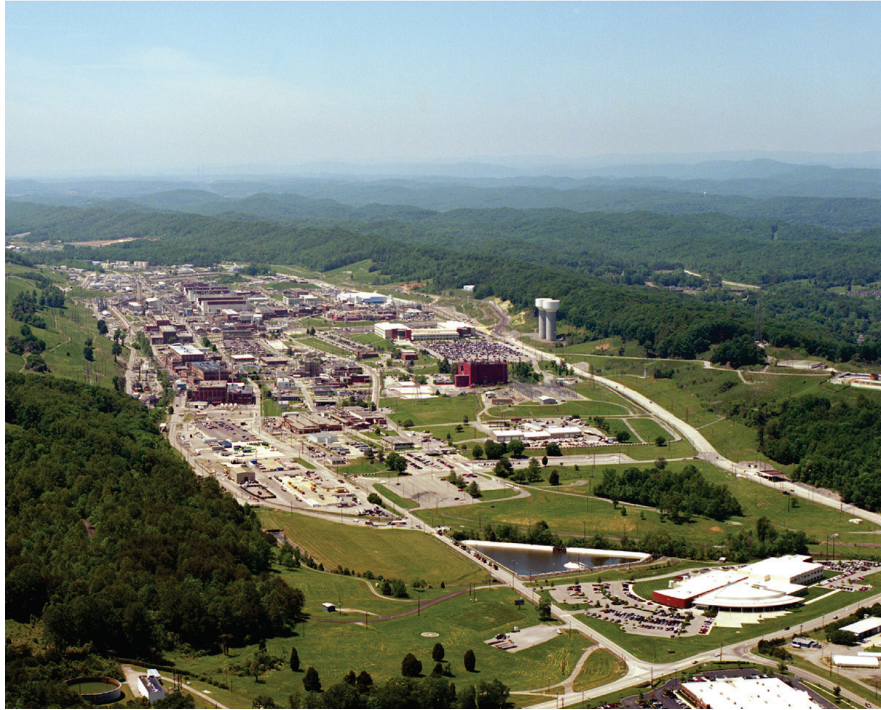
Fig. 1.8. Y-12 National Security Complex.
